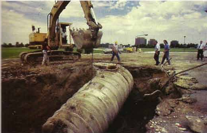
Excavated in 1990 after 26 years of continuous use in underground fuel storage (left), this FRP tank based on isopolyester resin was brought up to current code by the addition of a second manway, recertified and reinstalled (right) by Owens-Corning with three new tanks at another site in 1991. Photos courtesy of Amoco Chemicals.
