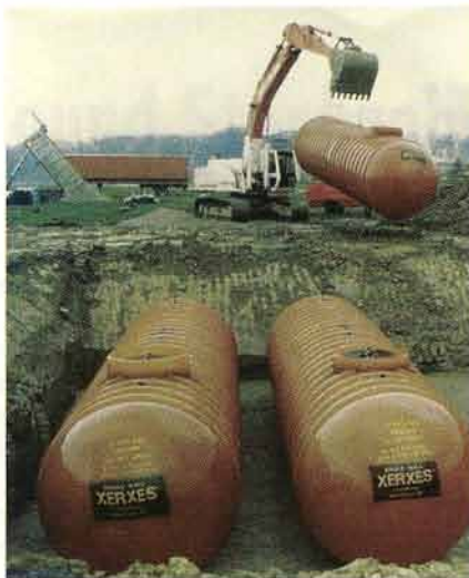
These single-wall, fiberglass, underground storage tanks from Xerxes Corp. are among the strongest, most robust tanks available due to a unique integral-rib design, and construction of resin and glass-fiber reinforcement.
