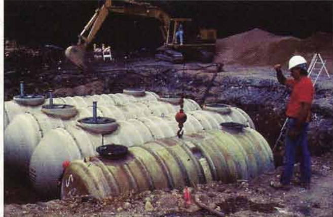
Excavated in 1990 after 26 years of continuous use in underground fuel storage (left), this FRP tank based on isopolyester resin was brought up to current code by the addition of a second manway, recertified and reinstalled (right) by Owens-Corning with three new tanks at another site in 1991. Photos courtesy of Amoco Chemicals.
